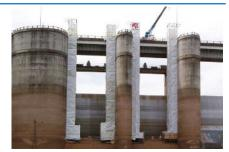
Dam wall was extended in 1991. Steel guide rails in the upstream face facilitate the installation of stoplogs allowing maintenance of the four radial gates.
