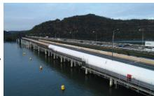
Scaffolding and encapsulation of spans, Abrasive blast lead abatement, Application of RMS 3 coat system. Concrete repairs, Cathodic protection, Steel repairs and installation of new crash barriers.
